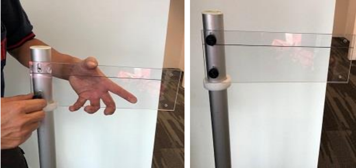
Fixing the acrylic panel
